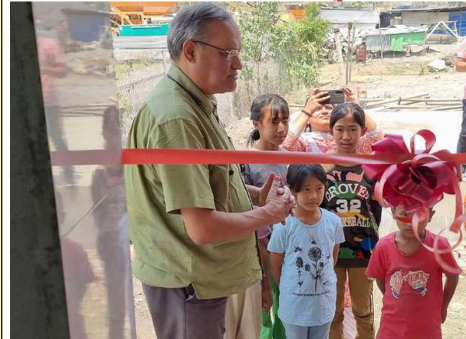
A newly-built toilet block, sponsored by Prestige Group , was inaugurated at Yapaal Friendship Hostel in Kakching, Manipur, by Col. Christopher Rego, Founder of Sunbird Trust. The new toilet block consists of 4 toilets and 2 bathrooms.
