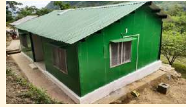
Staff quarters-turned hostel for 40, constructed by the Indian Army! Enrolment increases to 95.
